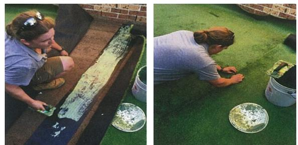
**5. JOINING** | Roll out the joining tape and pin at both ends to prevent it from moving. Trowel on synthetic grass adhesive glue then join the grass back together. Run a pin roller up and down the join to ensure the adhesive makes contact with the backing.
