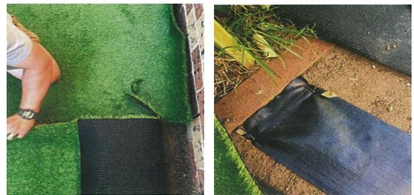
**4. MEASURE TWICE** | Trim off any excess synthetic grass overlay and if need be an extra stitch off the edge of the grass to ensure a straight edge. For a seamless join align the pieces with the stitches running parallel to each other equal distances apart. Joins done end to end may be visible. Also ensure the grain or direction of the grass on all pieces are running the same way.
