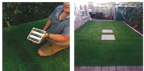
**6. SANDING** | Trim in edges with sharp knife, then broom the grass to make the blades stand upright. Evenly spread out the specified amount of kiln dried sand for your product (a sand spreader is useful on large jobs) and broom in properly.
